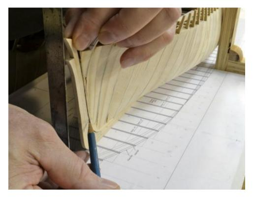
This allowed the forward deadwood to be trimmed to match the stem while the stem was removed and safe from damage. The next picture shows the fairing to the stem sides.
