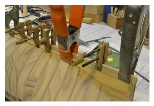
Because this strake twists to fay against the curving hull, a lot of clamps were needed. The next picture shows the aft section after the piece of second strake was installed.
