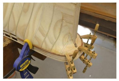
Screw clamps were used for this piece. It is not only curved around the stern but also twisted to be horizontal and not tilt downward. Straight-grained maple was used for all the bottom planking. Its flecked grain will be hidden by paint and metal sheathing. You will note in this picture that the topside planking above the planksheer was not yet installed. This would, of course, be installed before extending the rail forward.
