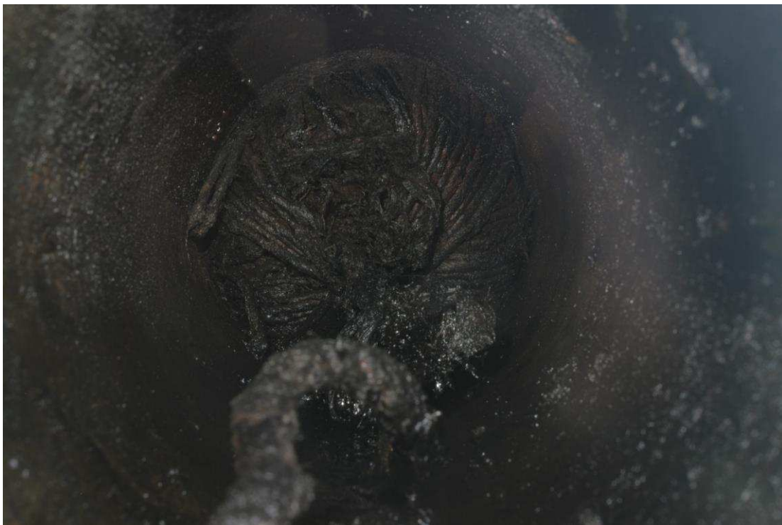
Figure 53. Ball of twine inside bore of ACC Oregon Carronade A. (Bajdek 2012)
