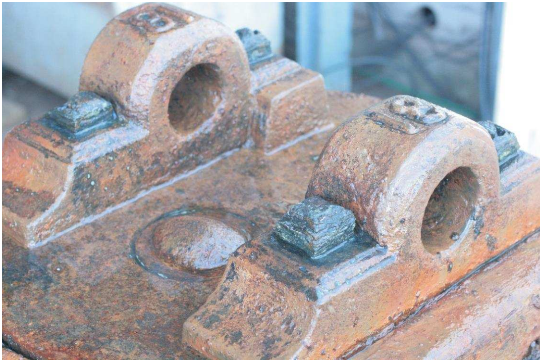
Figure 35. Joint chock with chock fastening bolts and molded 18 pound designation. (Bajdek 2012)
