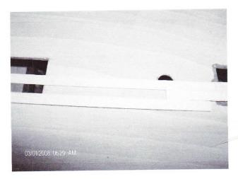
Step 3.- OK. So far so good. According to our pattern 1 3 5 2 4, to the right of the 5 plank, we will have a plank starting on line 2, and to the left, a plank starting on line 3. We will proceed as follows:
