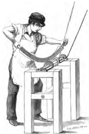
BEVELING RIBS OF NATURAL CURVE.
