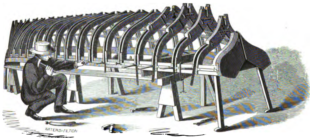
SECURING HEADS OF RIBS ON FORM.
